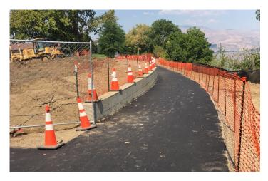
8-7-2024 The new configuration for the Loop Trail isn't finished, but is in place (above and right) just north of the Riverfront Crossing junction. Two temporary fences on the river side of the trail will eventually be replaced by a sturdy fence along the edge of the bluff.
