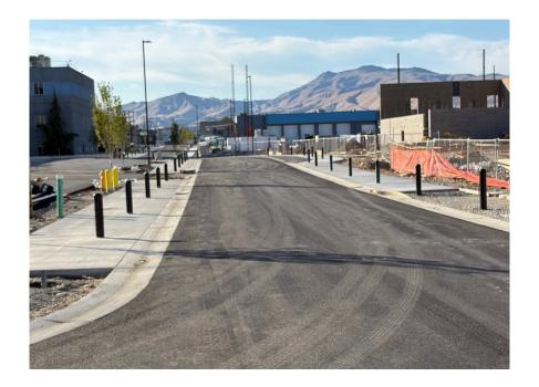
Electric Ave (left) is a new kind of road in Wenatchee that is designed for slow speeds, so it should work well for bicycling. When the road signs are finally placed, the speed limit will be 20 mph. Sidewalks are without curbs, so bollards are placed to keep motor vehicles off the sidewalks.
